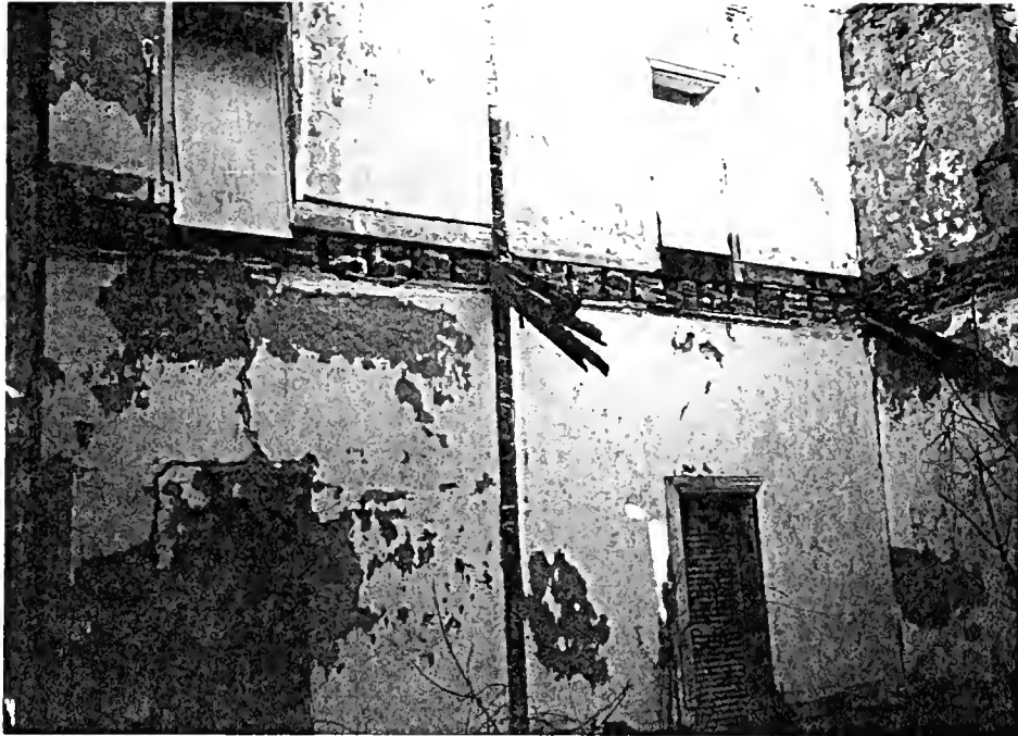
Figure 35: Northern interior wall of addition (connected to Pawling portion of house)
